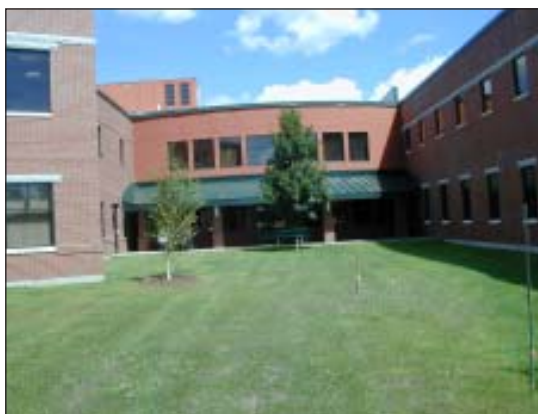
Connector Between Existing Building & New Addition
