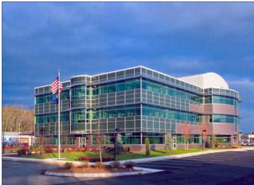
Exterior Southwest View
