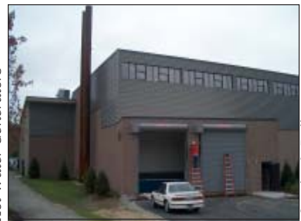
Stacks & Delivery Bays
