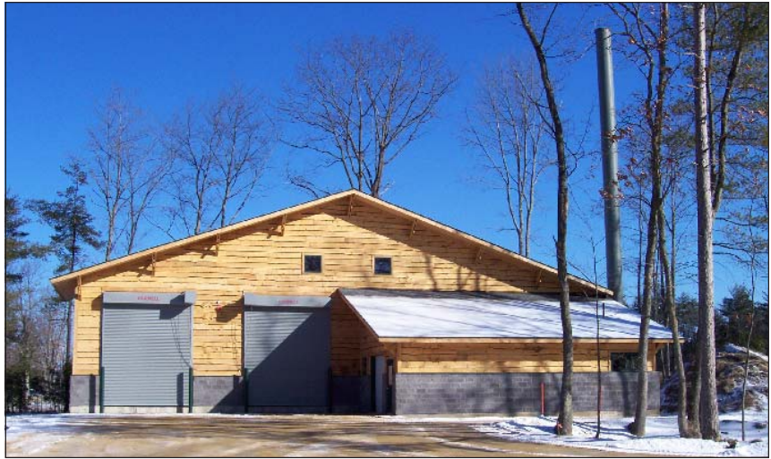
Merrimack Valley Woodchip Plant
